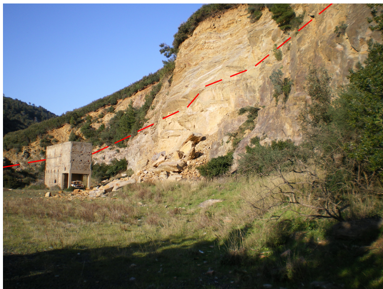
Fig. 4. The red line (OFBS) divided an open fractures zone (over the line), from a mineralized fractures zone (under the line). Quarry of Rio Calignia near Leghorn.
